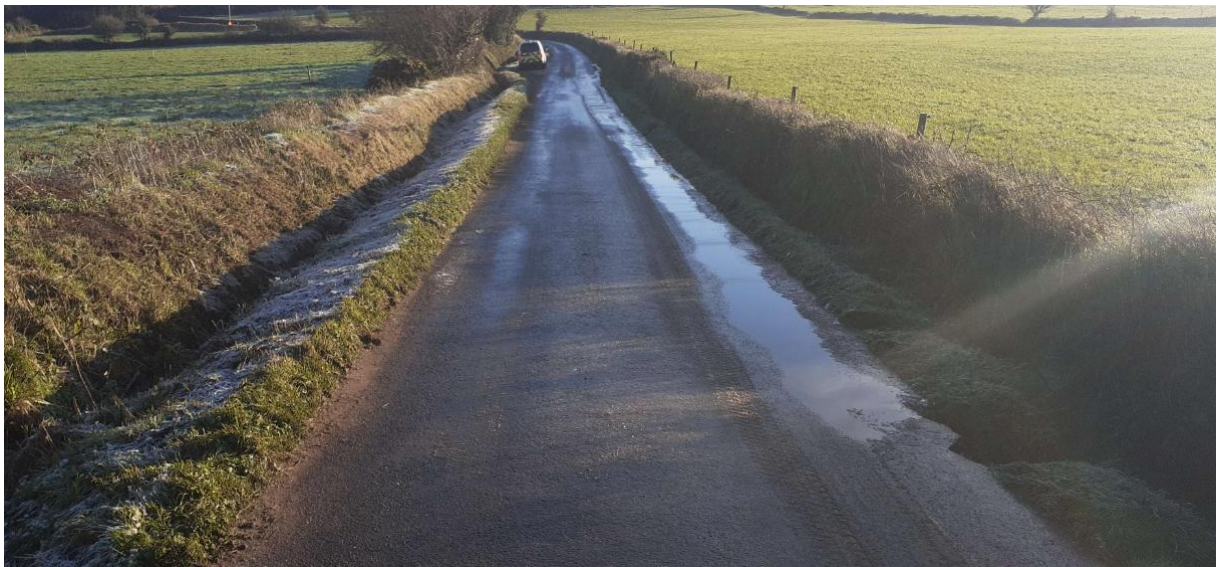
Figure 19 - Culvert position with L-1505
