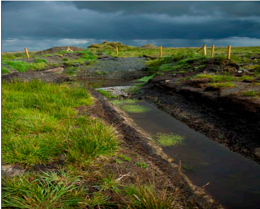
Figure 2: Swale draining to Settlement pond
