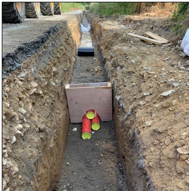
Figure 4 - Typical Single Circuit 33kV Ducting Installation
