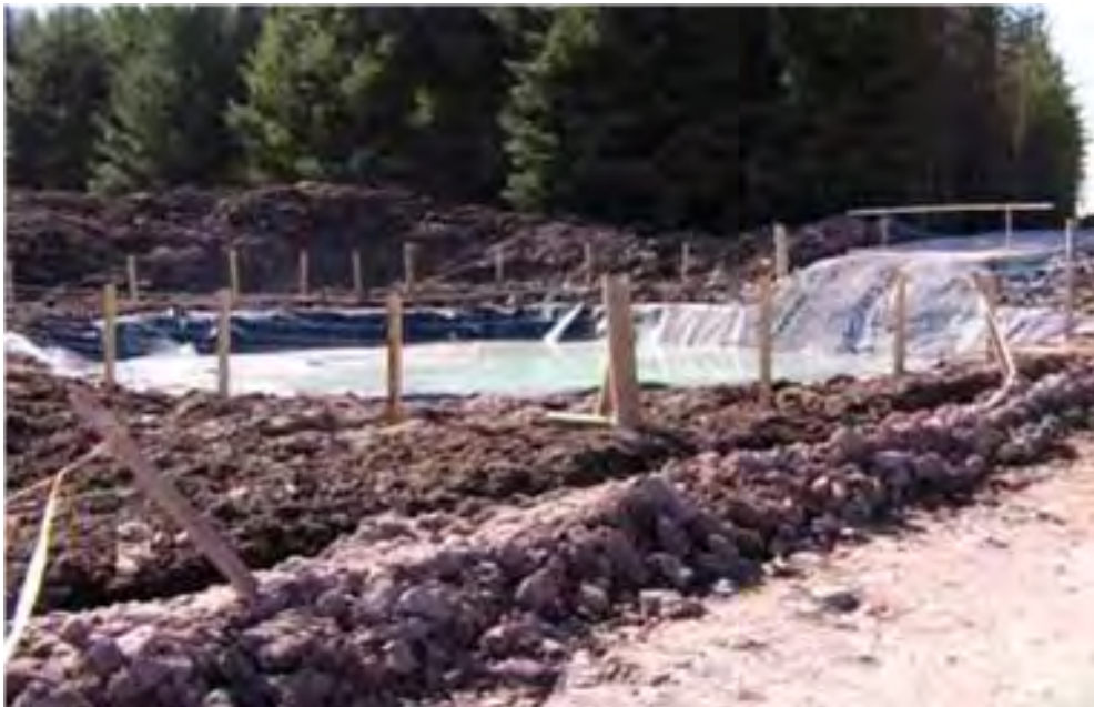
Figure 8: Lined Settlement Lagoon for Concrete Washout Facility
