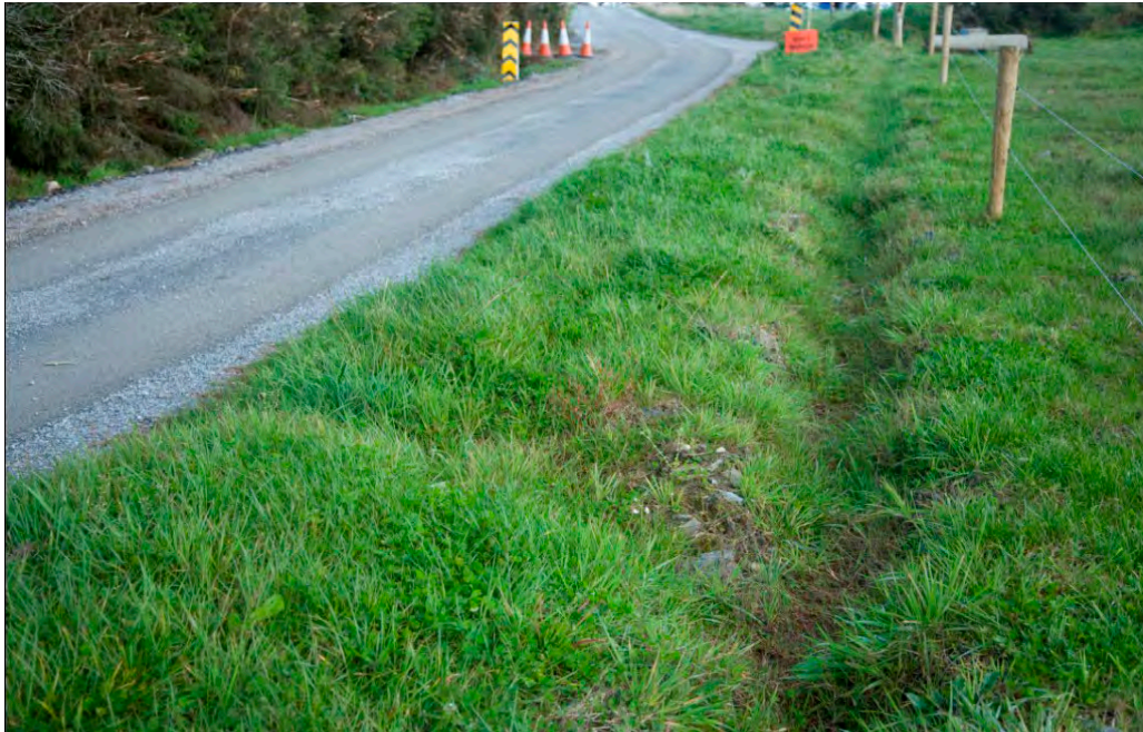
Figure 1: Grassed Swale along access track
