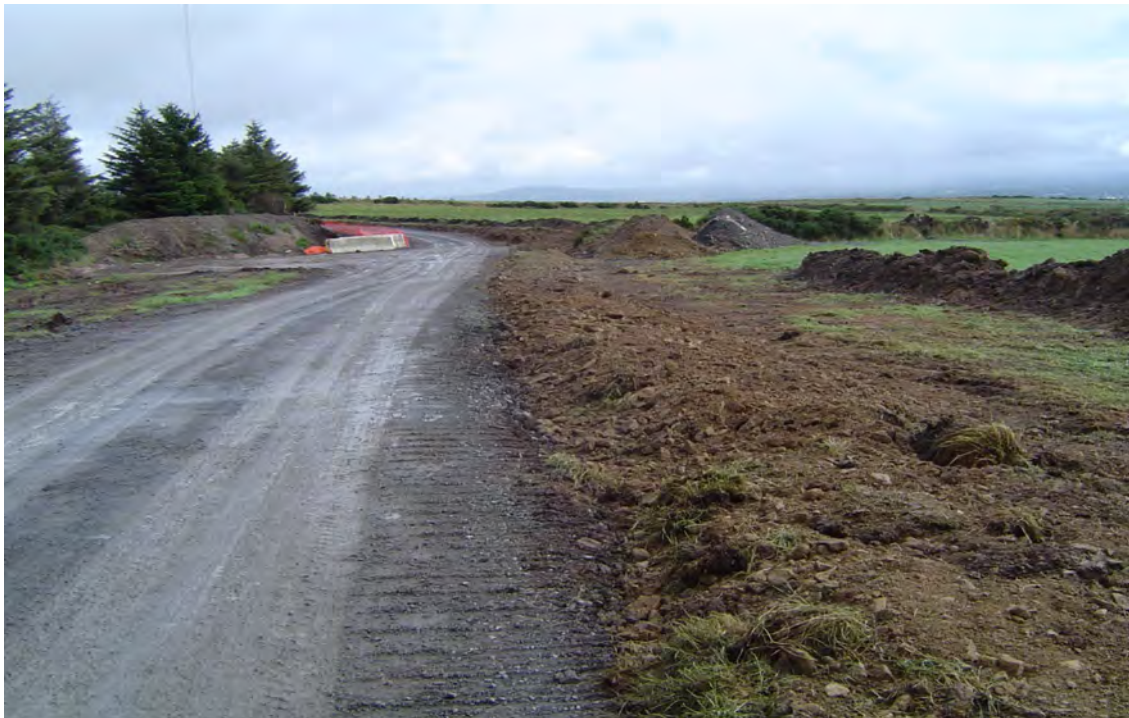
Figure 7: Backfill over Cable Trench
