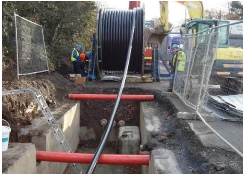
Figure 14 – Typical Cable Pulling Drum Set Up
