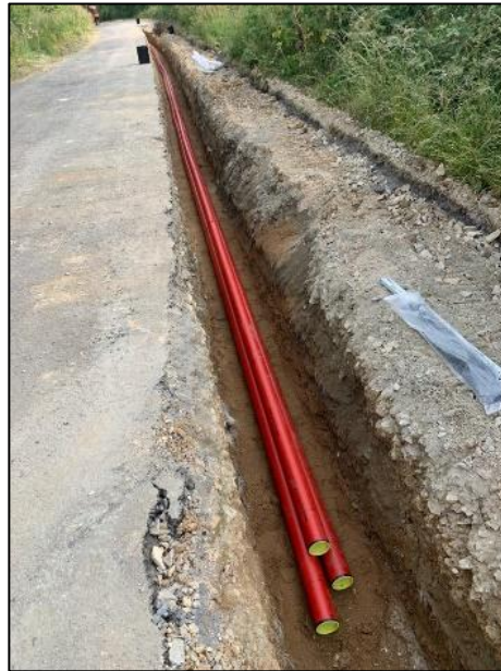
Figure 7 - Typical 110kV Underground Duct Installation
